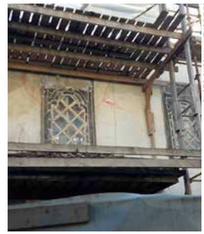
Images from the renovation of the Khan's Palace show destroyed original masonry and authentic ornaments.
